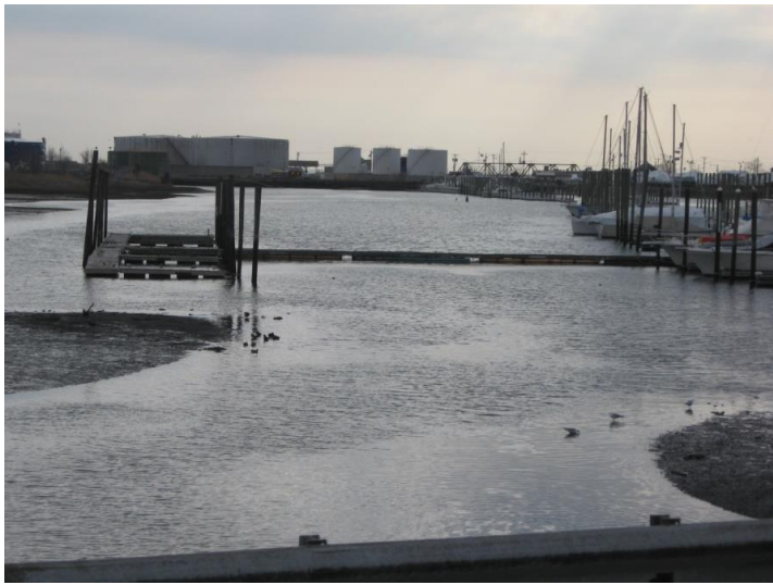
Figure B5.2. Looking down Johnsons Creek, which has many commercial land uses on its borders. The swing bridge in the background (now removed) is where Johnsons Creek meets Lewis Gut.
